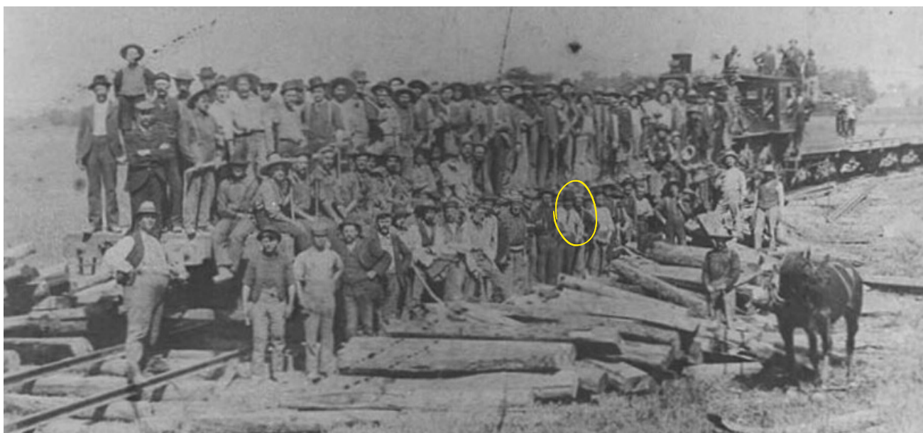
Last day of work on the Schomberg & Aurora Railway Line, c. 1902
